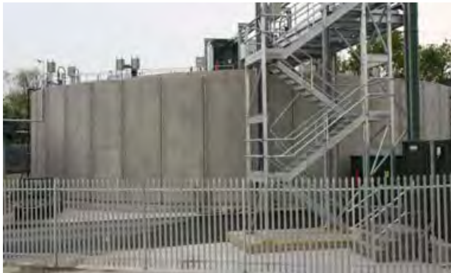
The wall of the tank built with concrete segments
